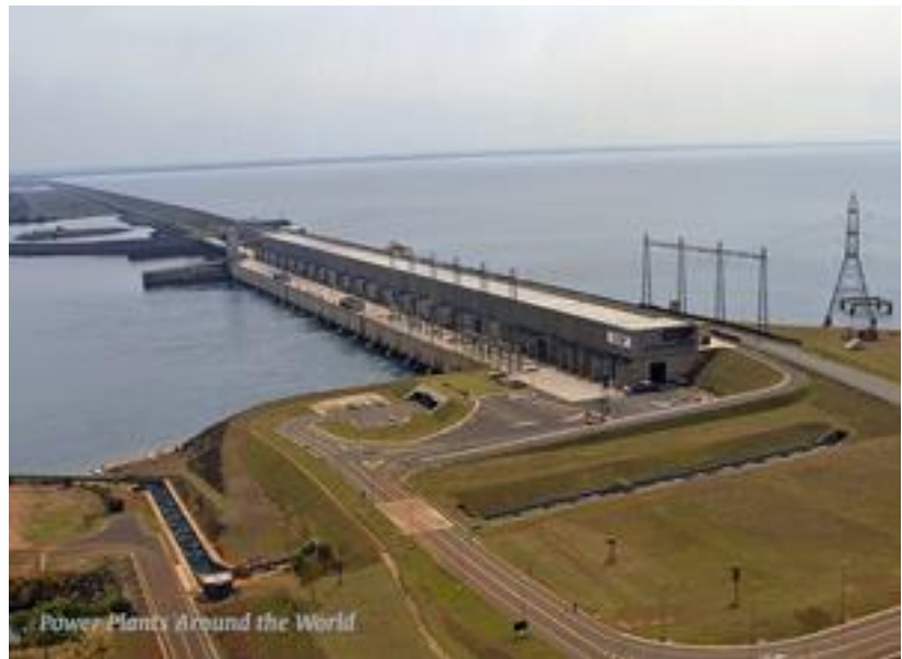
Figure 10 Engineer Sergio Motta Dam (Hydro Brazil)
