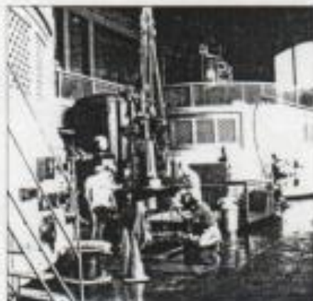
Replacing a governor at Philadelphia Electric's Conowingo hydropower plant.
