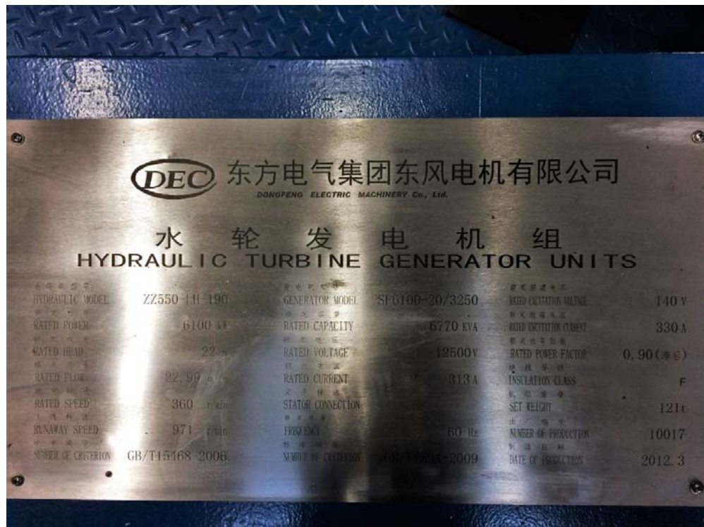
Figure 3-1: Kaplan Unit Turbine Name Plate
